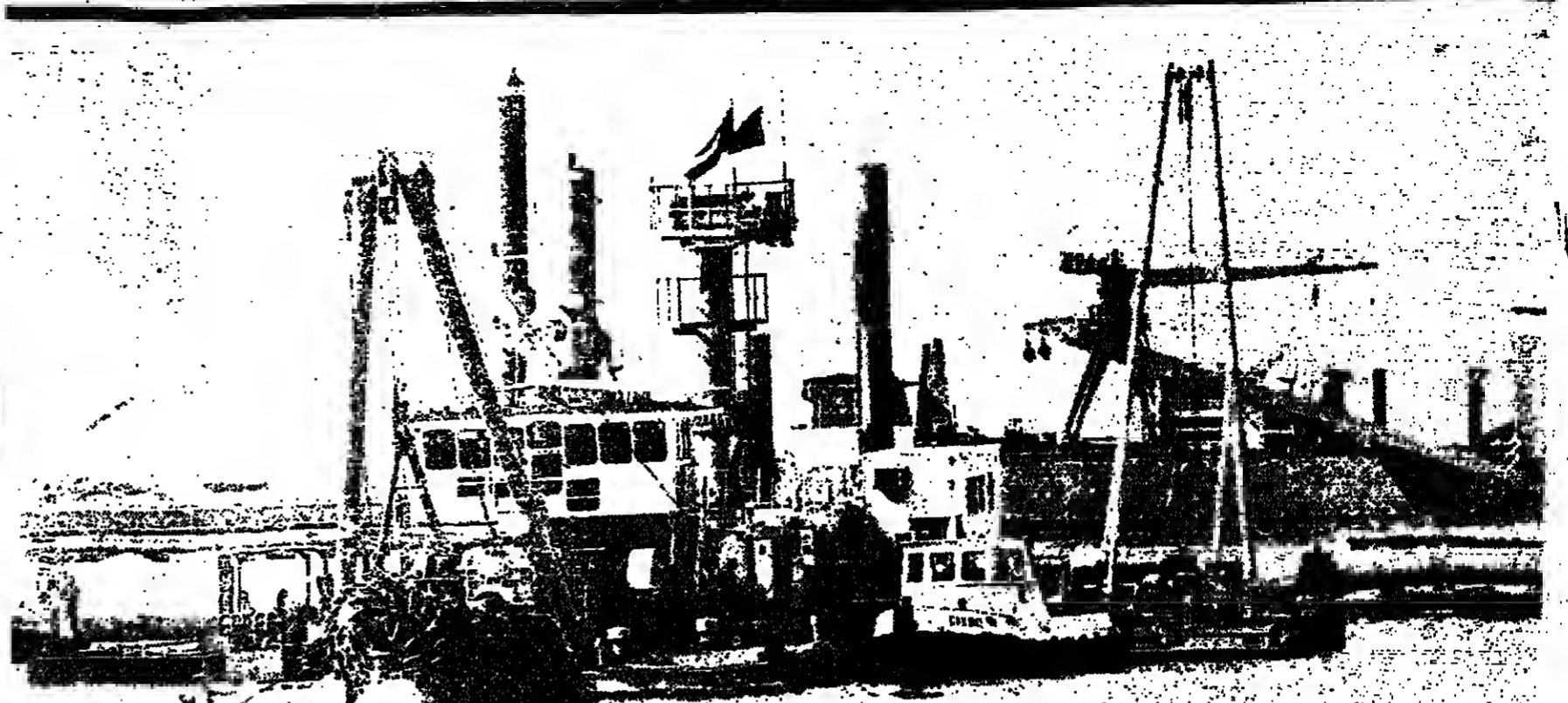
The £1bn port at Mina Jebel Ali is being constructed by Gulf-Cobra for the Ruler of Dubai. The two basins will have 66 landlocked berths and will be completed by February 1981. One feature of the construction of the 15km of dock walls is the use of special hydraulic tongs for the placing of quay wall blocks
